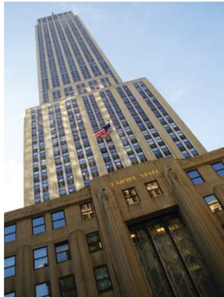
The Empire State Building: A sustainable retrofit has yielded huge savings on energy costs
